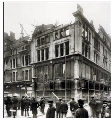
In 1912 Barkers was demolished by a fire, which also killed five staff.
