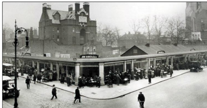
After the fire, a temporary building was quickly erected on the north side of Kensington High Street, housing the food department.
